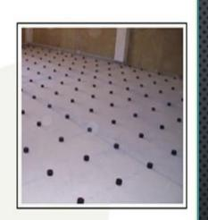
The EANF neoprene floor isolators all perform below 8.5 Hz. Compounding is to AASHO specifications and mounts are supplied by Enginias Inc., Canada
